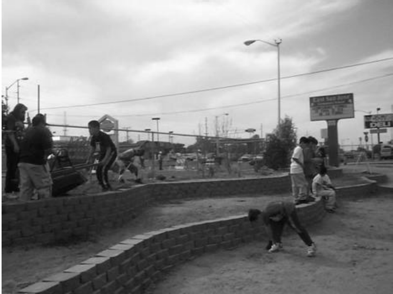
Further work on the serpentine terrace walls.
